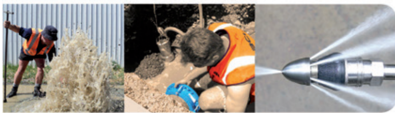
Pipe & Drain Repairs & Unblocking
