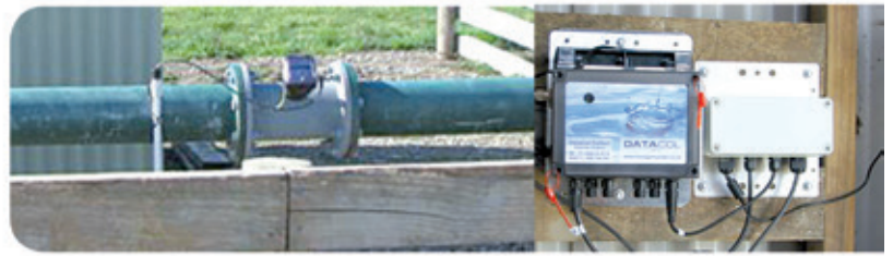
Irrigation Watermeter Installation
